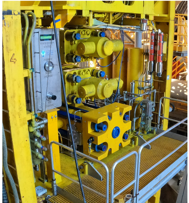
18-15M K-BOS retrofit installed in Cameron TL BOP stack
