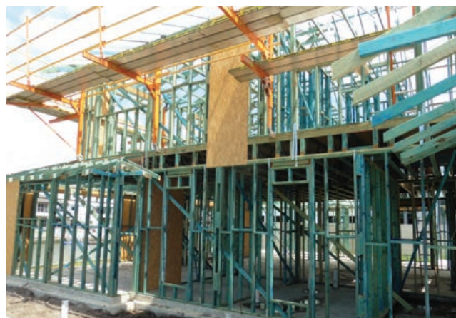
Termite resistant timber framing
