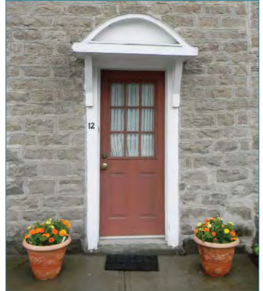
The retention of original features such as doors and windows is critical, as here in Spencerville. (Guideline 1).
