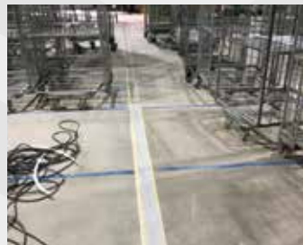
EXPANSION JOINT TREATMENT
