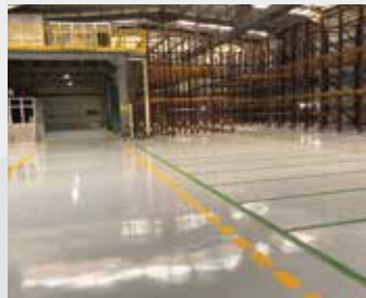
SELF-LEVELING EPOXY FLOORING
