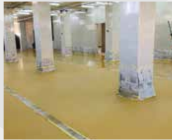
FOOD-GRADE FLOORING [POLYURETHANE SCREED FLOORING]
