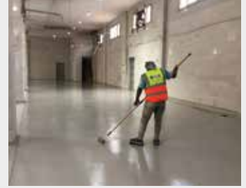
EPOXY COATING FLOORING
