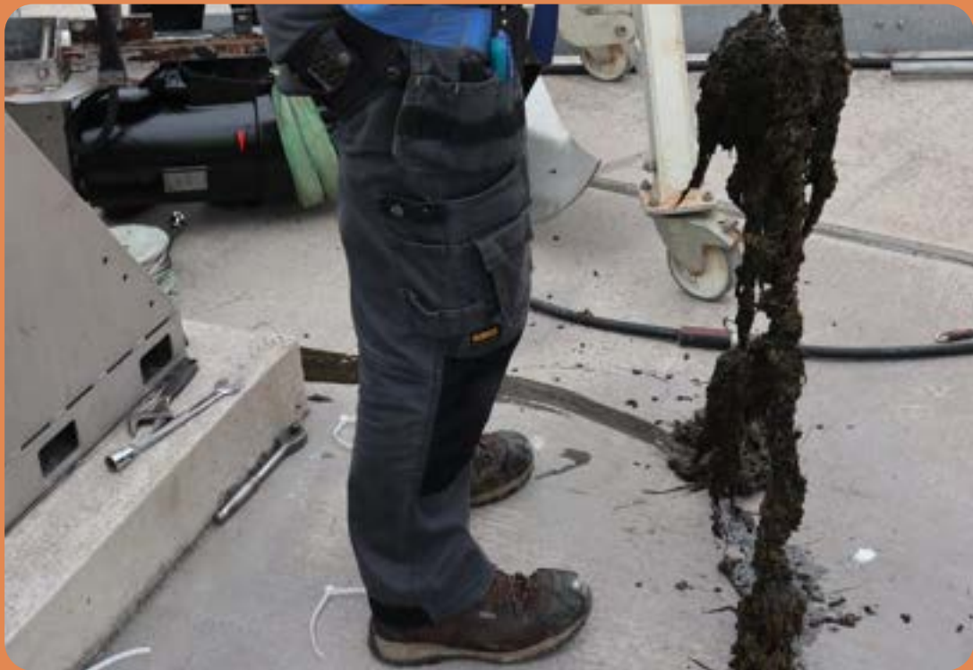
FIGURE 8: 'ROPES' OF UNDEFINED COMPOSTABLE PLASTIC MERGING IN A MESOPHILIC WET DIGESTER TO FORM A FLOATING LAYER
