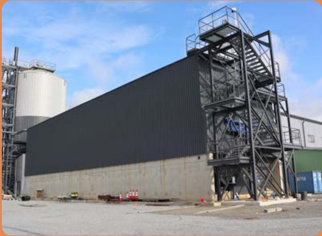
FIGURE 12: MUNICIPAL ORGANIC WASTE PRE-TREATED AND PROCESSED AT A HYBRID WET + DRY + IN-VESSEL COMPOSTING FACILITY IN NOKIA, FINLAND
