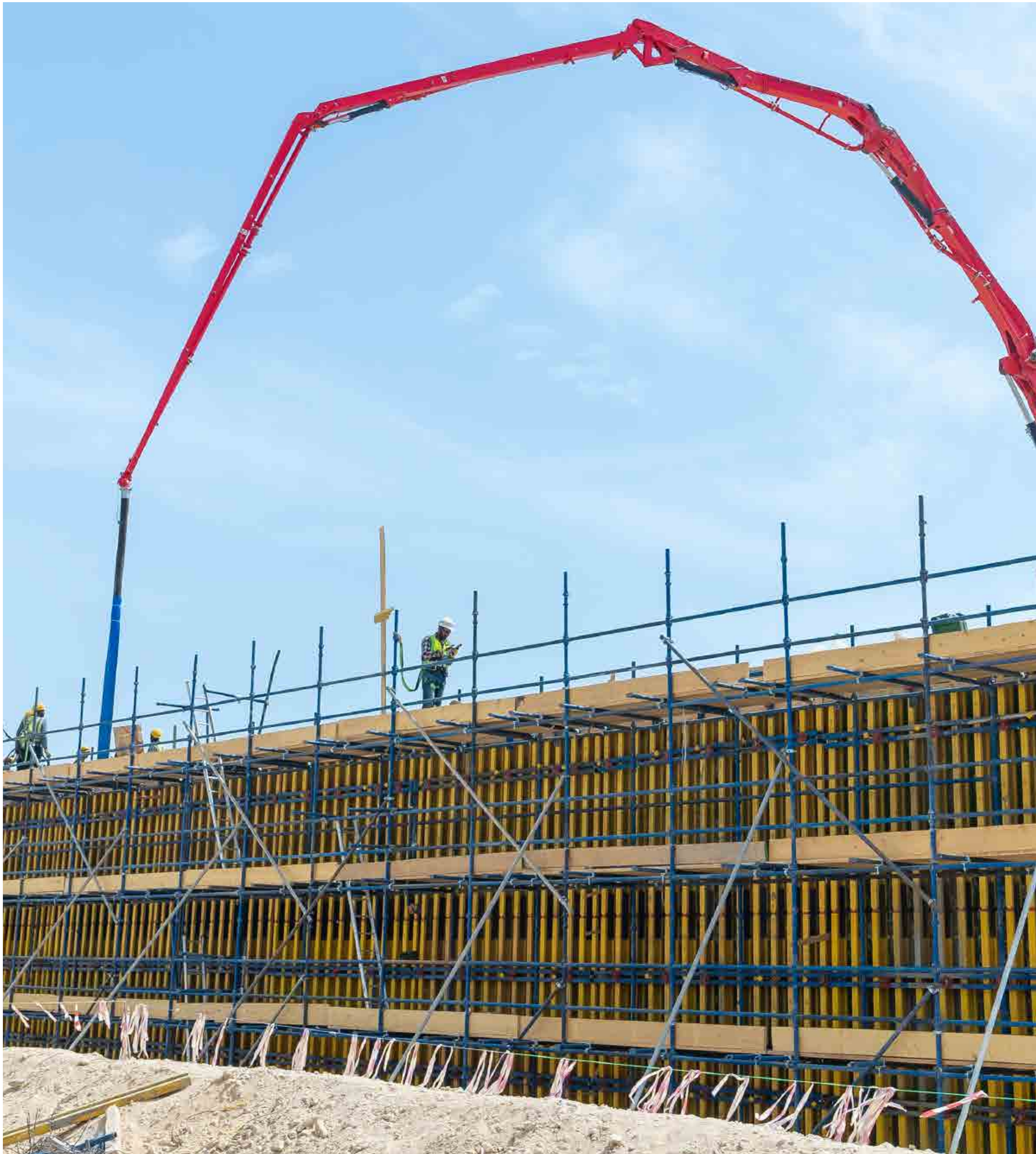
Utilizing concrete pump trucks for efficient pouring within the extensive formwork.
