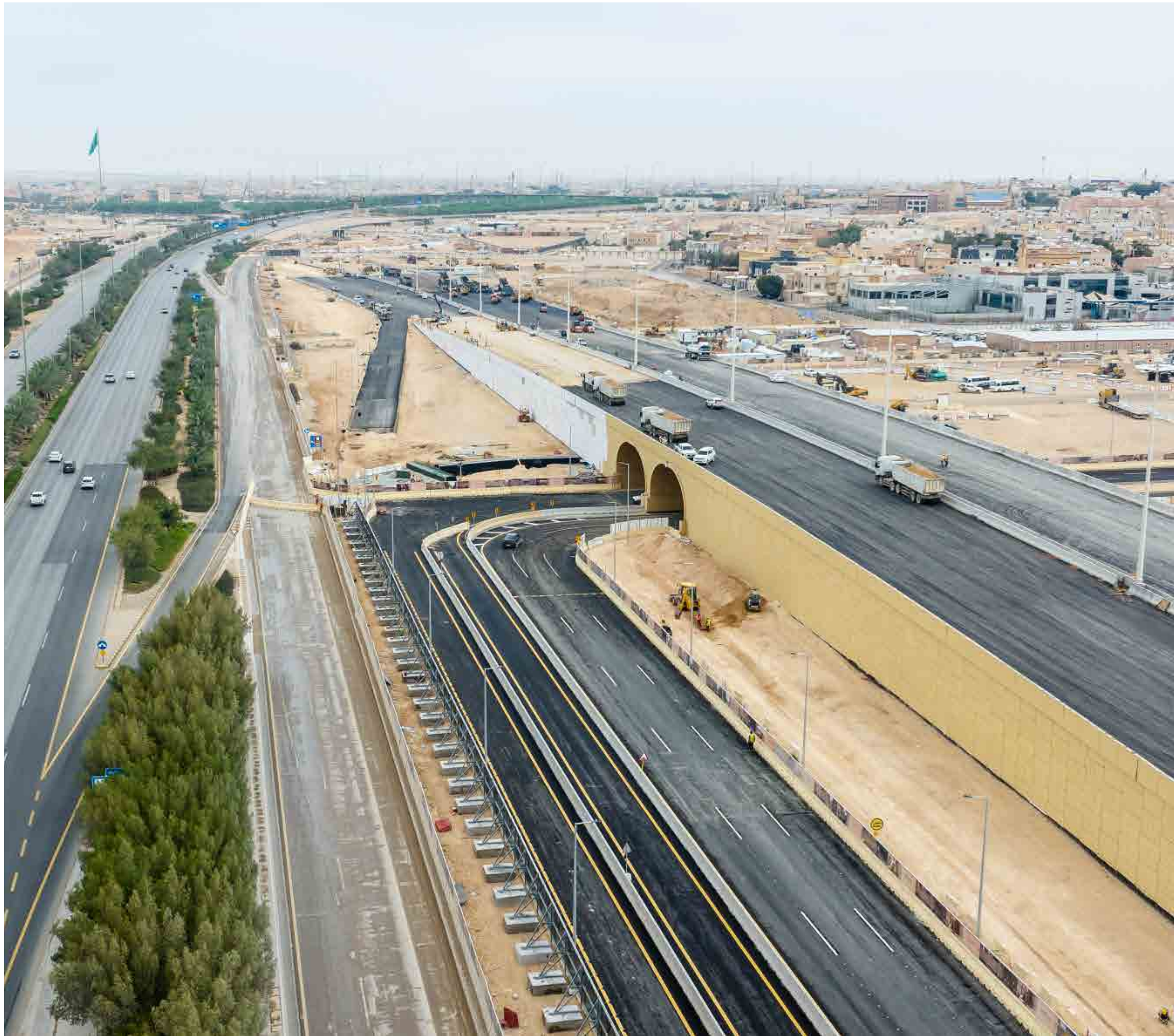
The main 3km carriageway flanked by 8-meter high MSE retaining walls, connecting to the underpass structure.
