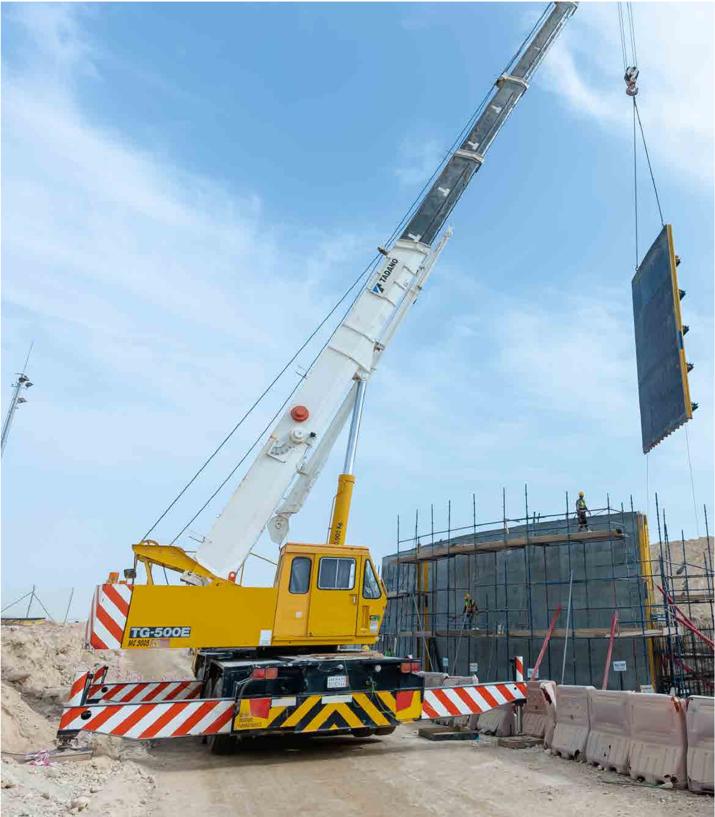
Heavy crane lifting and placing large formwork panels for the concrete retaining wall construction.
