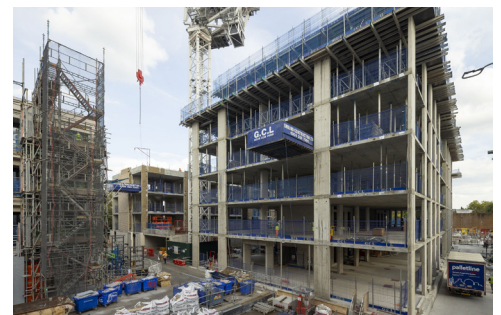
Concrete frame for Building 6 (centre of site)
