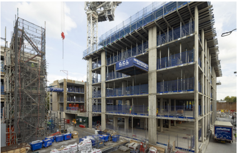
Concrete frame for Building 6 (centre of site)
