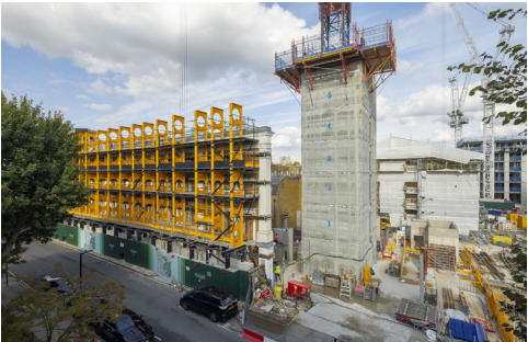
Core and façade retention for Building 9 (Queen's Terrace)
