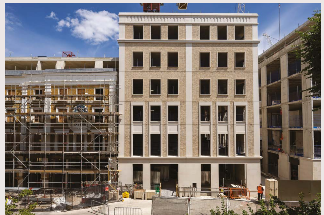
Progress at Building 9, Queen's Terrace
