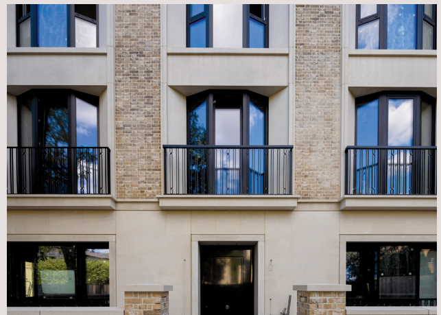
Building 5, Ordnance Hill – Completed façade
