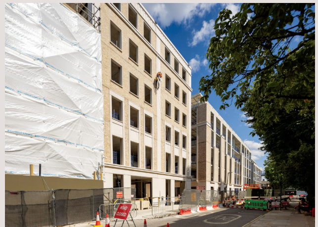
Building 9, Queen's Terrace – Façade Installation in Progress
