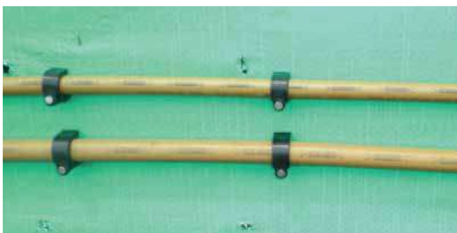
Figure 14.3 Install piping services prior to the installation of STAAC WALL® panel
