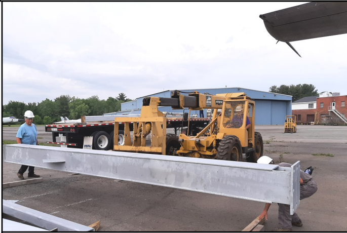
1. Receiving the Steel
