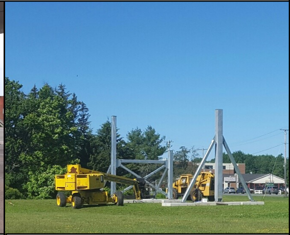
2. Erecting the Steel
