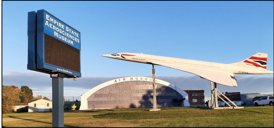
The Front of ESAM's Main Hangar has been redone in White and Blue-Gray. It looks great!
