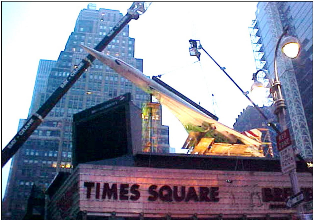
Concorde suspended by cranes while being detached from its supports
