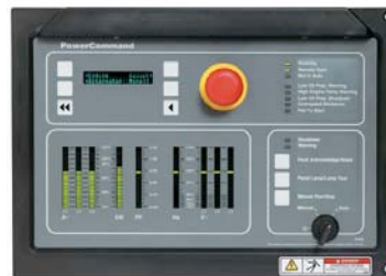
PowerCommand 2100 control operator/display panel
