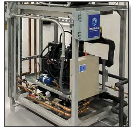
OverShield installed on a refrigeration skid
