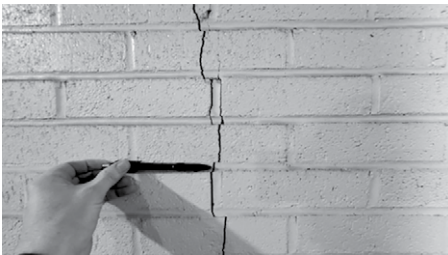
Cracked brick on inside wall of truck garage
