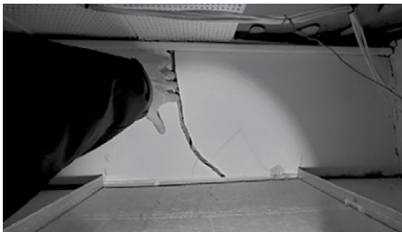
Cracked ceiling
