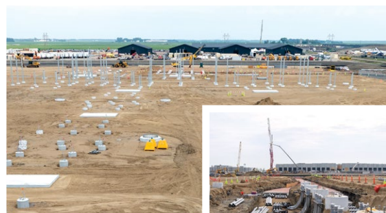
Construction continues on the Applied Digital data center near Harwood, North Dakota.
