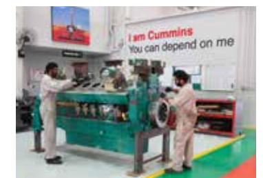
GENERATOR & AUXILIARY MAINTENANCE
