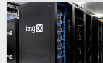
Loss of Critical Systems
