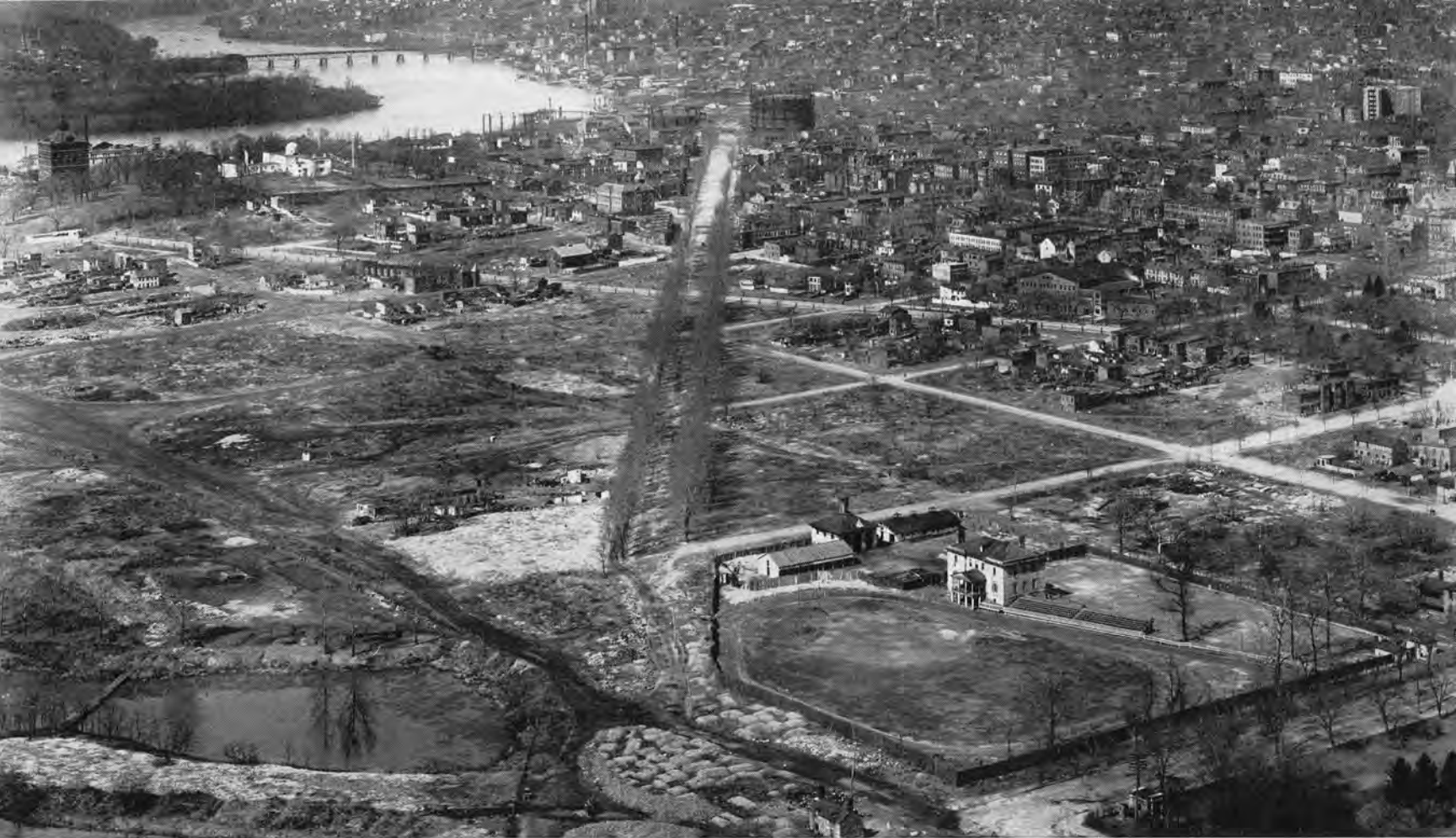
An early view from the Washington Monument showing the West Station Gas Works. The original buildings were constructed in 1858. The Pan American Building occupies the site of the race track in the foreground.
