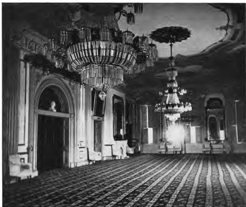
Earliest photograph of East Room of Executive Mansion, showing gas-lighted chandeliers. Photo by Brady in Lincoln's time.
