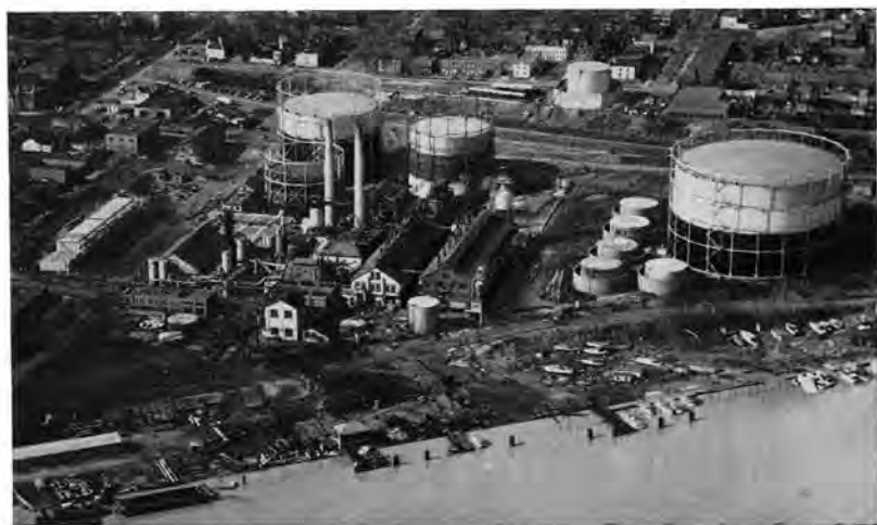
East Station Gas Works. Original buildings were constructed in 1888.
