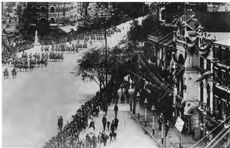
Pennsylvania Avenue around the turn of the Century, showing parade of the National Jockey Club. Four gas lamps can be seen in front of the Globe Theatre.
