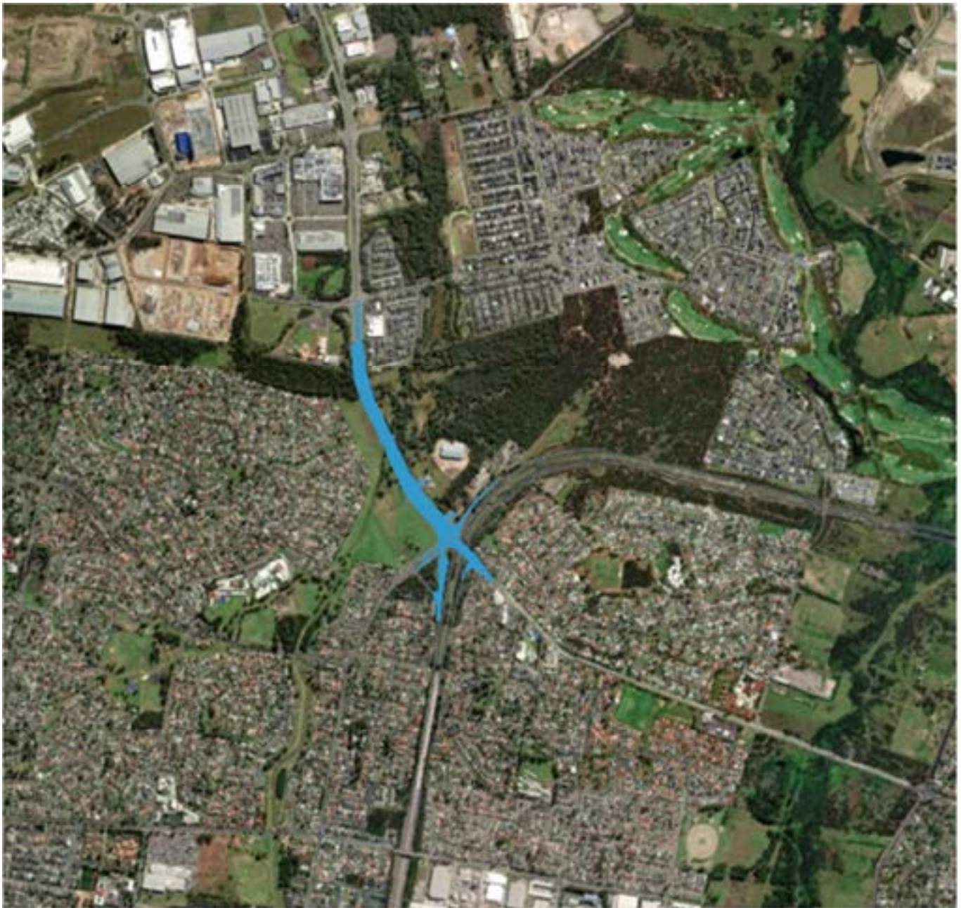
Figure 1-1 Project site overview
