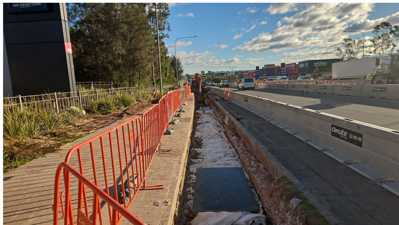
Drainage works in Zone 4B
