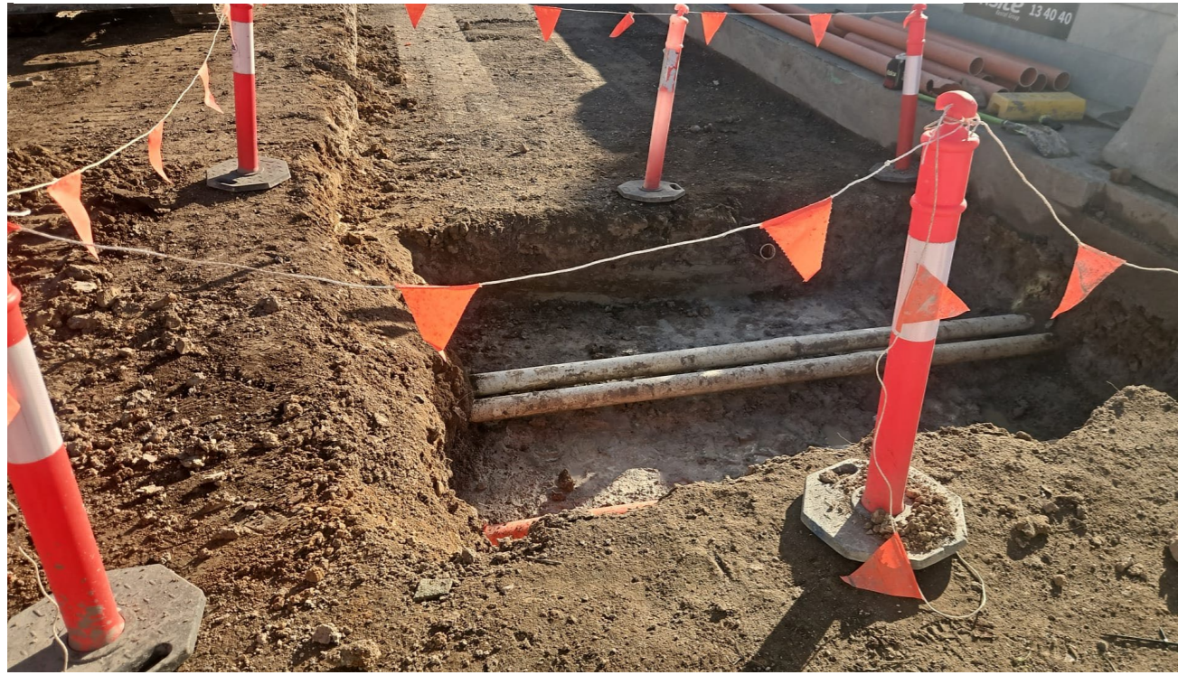
Pavement works in Zone 3
