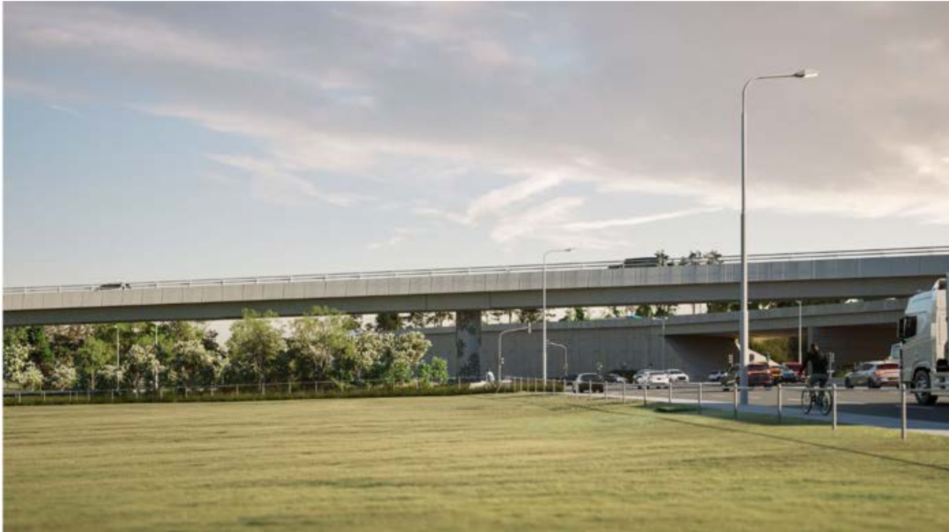
Figure 16: Visualisation of the Flyover bridge from the BNI site (all artwork is indicative only)
