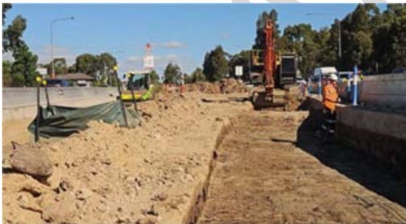
Figure 6: Example of temporary traffic barrier setup
