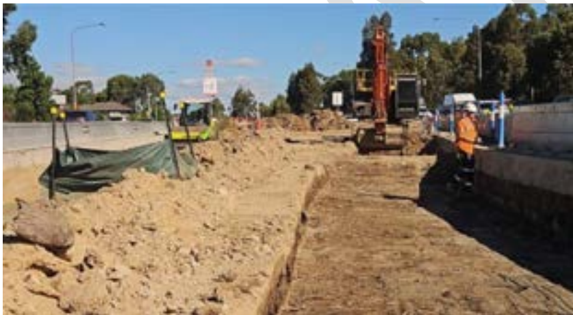
Figure 6: Example of temporary traffic barrier setup
