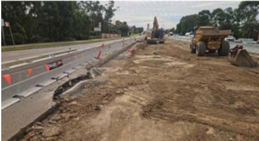
Figure 7: Example of pavement removal and temporary barrier set up
