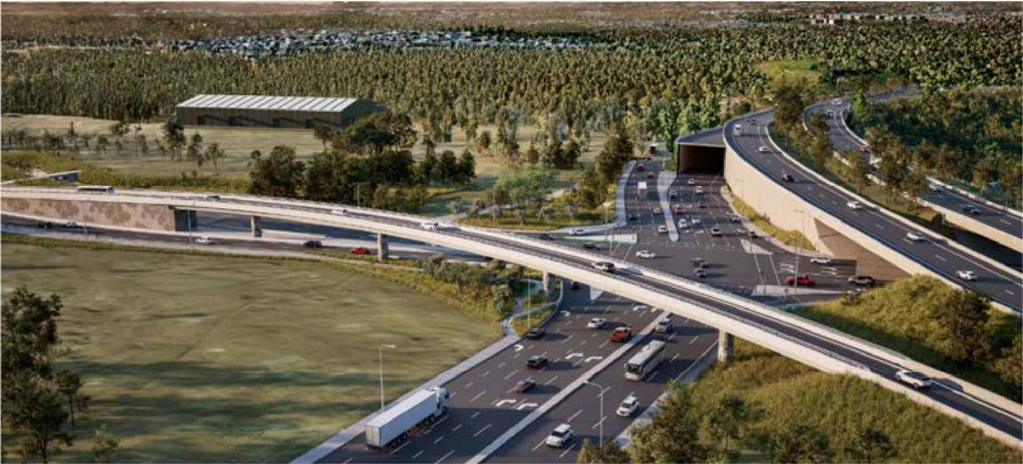
Figure 14: Visualisation of flyover and retaining wall, with landscaping and road works on Richmond Road (shown at 5 year maturity)
