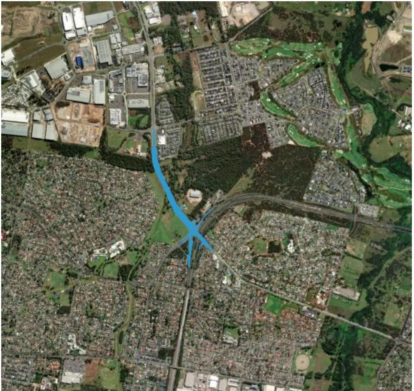
Figure 1 Project site overview
