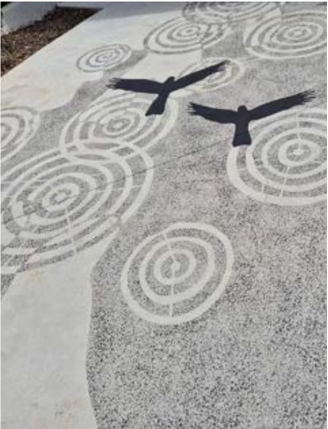
Figure 20 Sandblasted and painted concrete along the Medlow Bath Pedestrian Bridge
