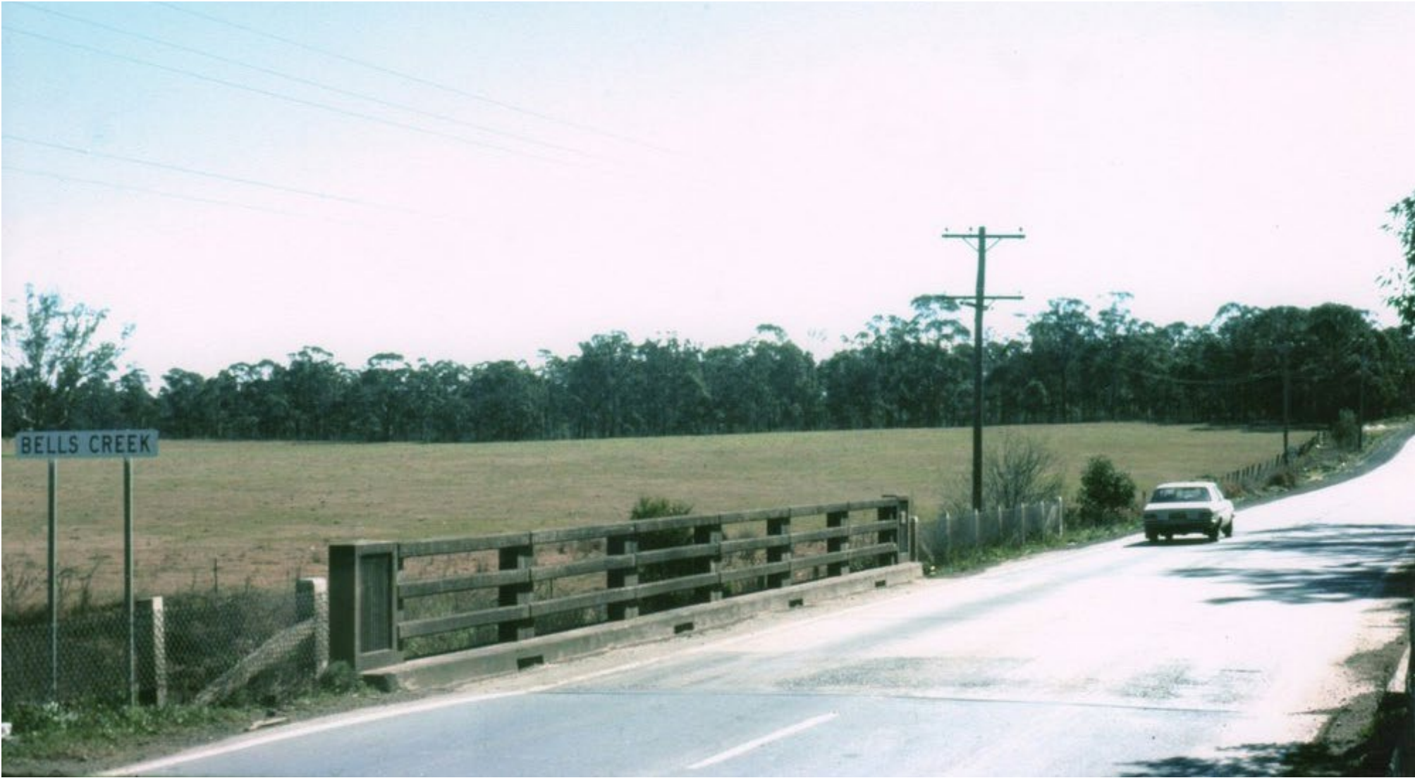
Figure 12: Richmond Road crossing Bells Creek, 1960
