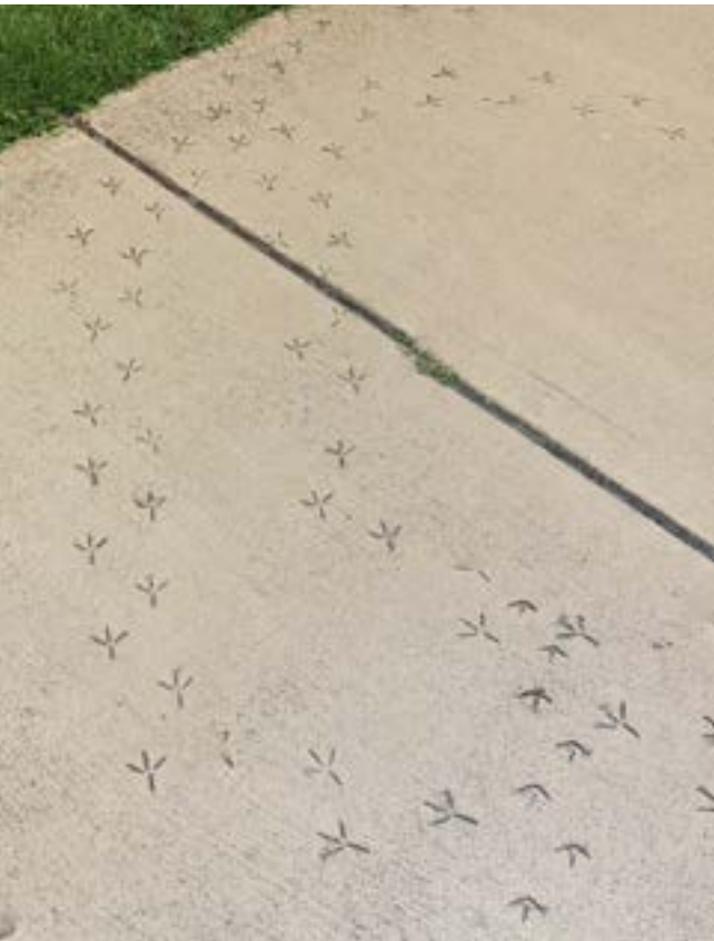
Figure 17 Imprints in concrete along the Woolloowara shared path, Sutherland Shire Council
