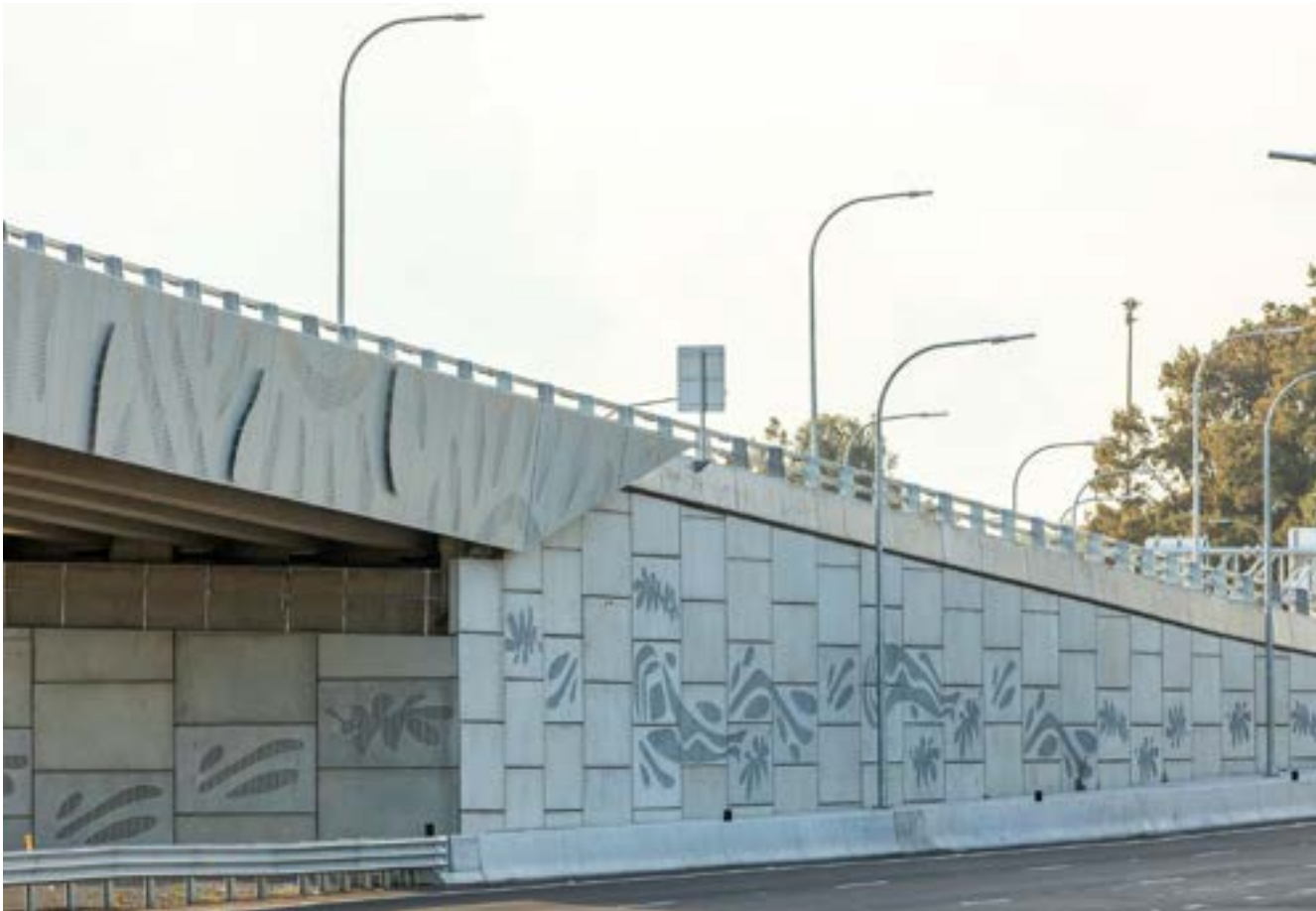
Figure 6 Photograph of the Sydney Gateway Project featuring artwork by Dennis Golding on the walls. Source: Cultural Capital, photograph by Aran Anderson
