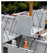
Precast concrete panels
