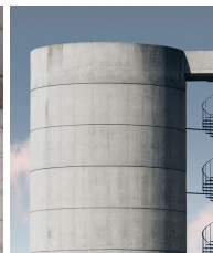
Concrete Tank Lining
