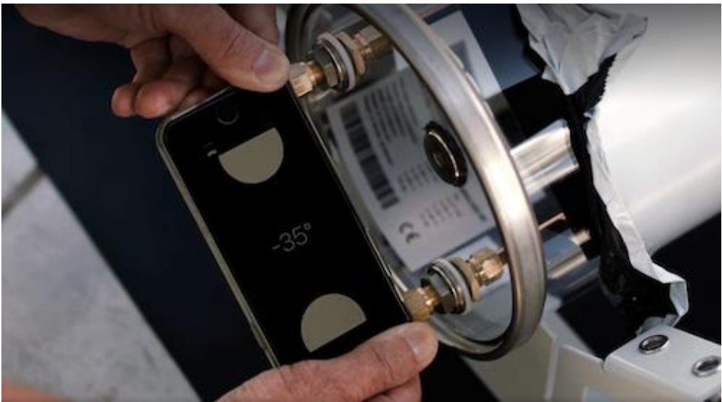
Figure 26 - Tube Angle is pre-set to 35° for flat roof installations
