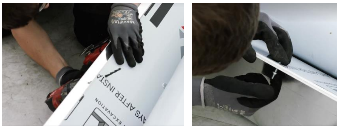
Figure 10 - m8 Nut and Bolt used to fix both Reflectors to each other
