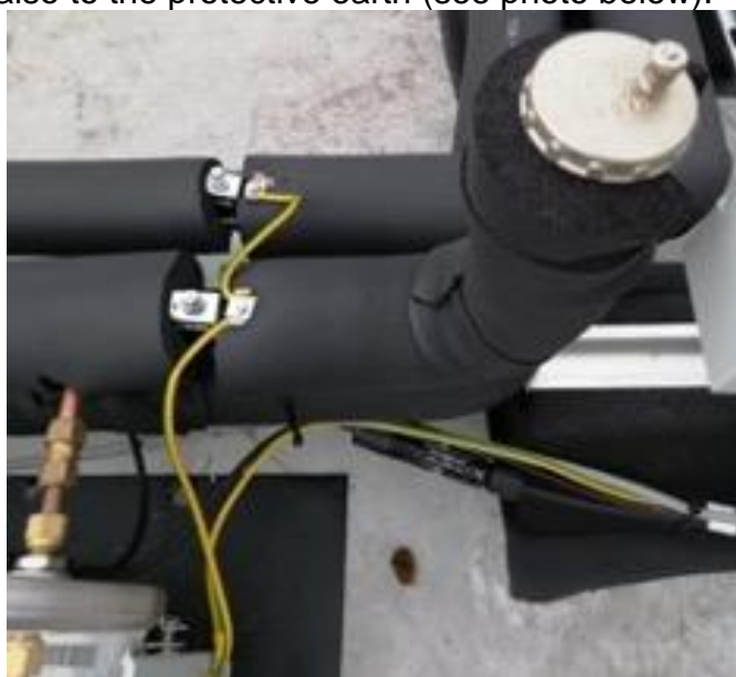
Figure 11 – Earthing/Bonding
