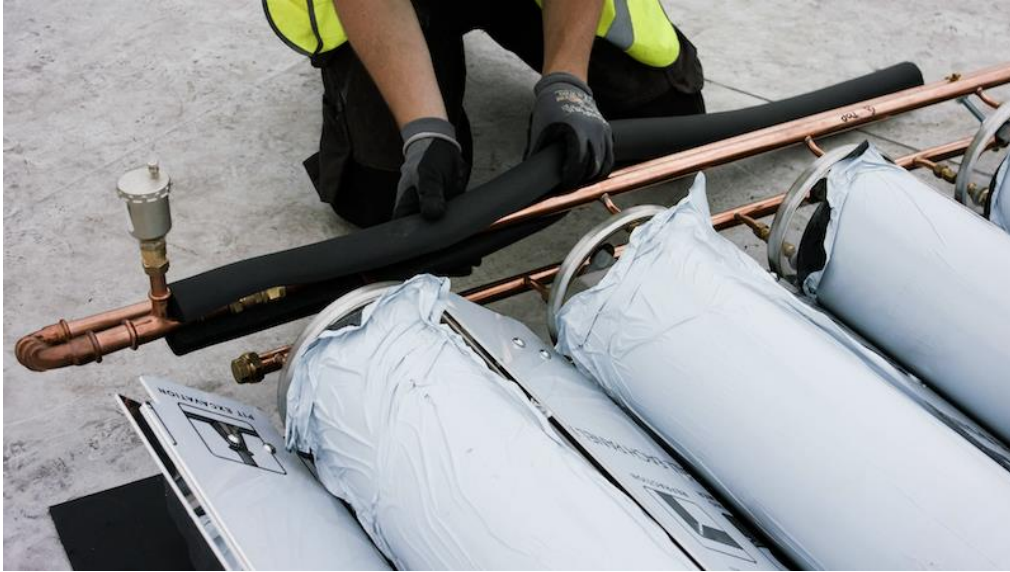
Figure 2 - Fitment of UV Rated Insulation
