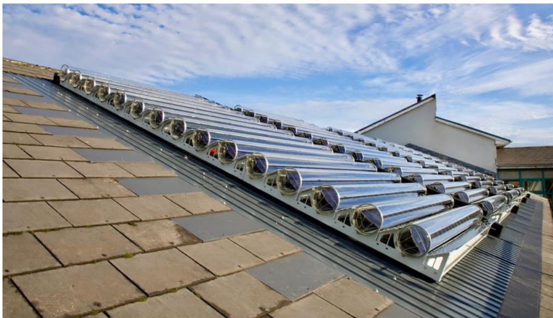
Figure 9 - 60 Virtu Tube Pitched Roof Installation in parallel
