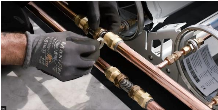
Figure 35 - Fitment of Flexible Connectors between each bank in series
