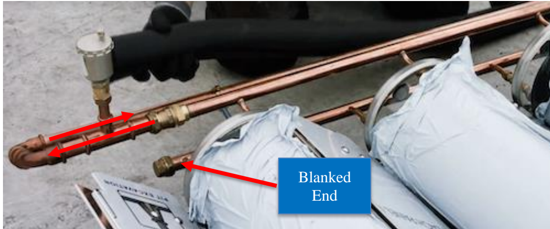
Figure 3 - Return to Plant Room from Hot Return pictured along with Blanked End on Cold Feed
