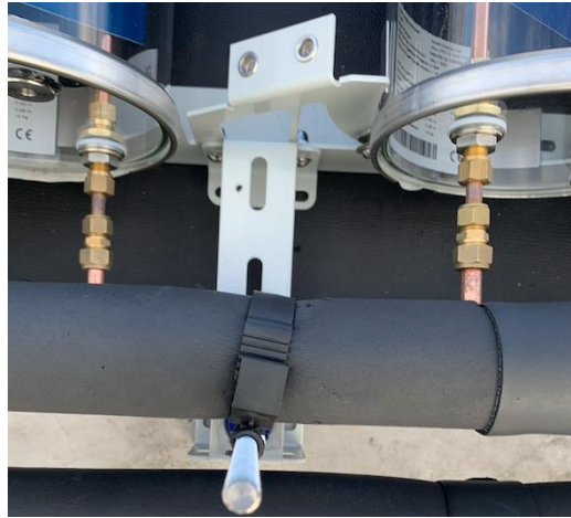
Figure 5 - Manifold Support Bar and Strap
