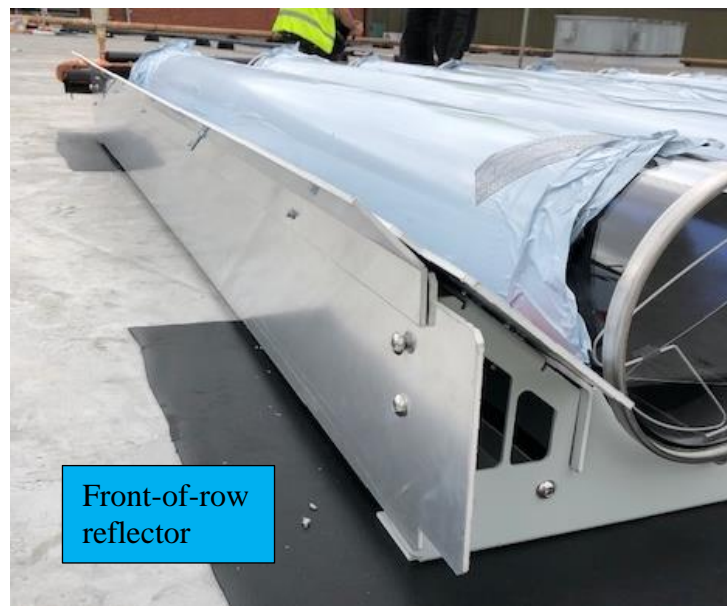
Figure 9 - Reflector fitted to support the underside of the End of Row Reflector
