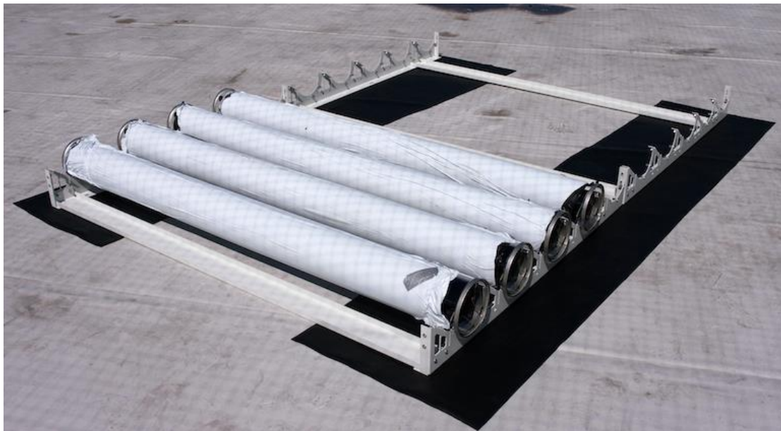
Figure 7 - 2 x VirtuHot Frames connected in series during installation
