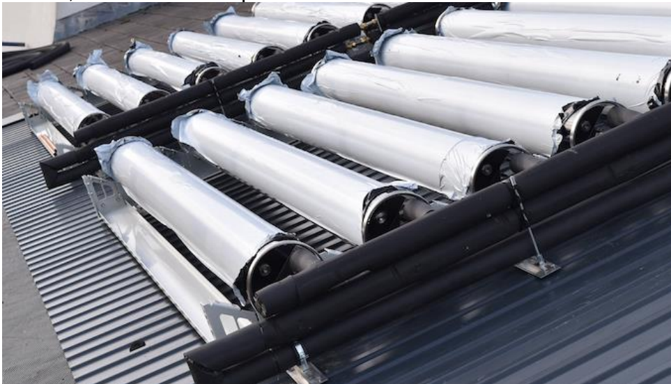
Figure 4 – U-bend Manifold Routing
