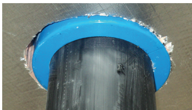
Figure 7 Penetration example - Kingspan Kooltherm® K10 G2 Soffit Board installed tight around the fire collar and HDPE service pipe.
