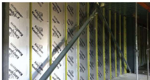
Figure 6 Side elevation of Kingspan Kooltherm ® K12 Framing Board clip-and-channel system
