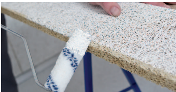
Painting the bevel - Use a brush or a thin paint roller to apply the paint.
