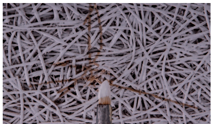
Chipped fibre - Cover chipped fibre with a fine brush or a spray gun using the supplied paint or an equivalent.
