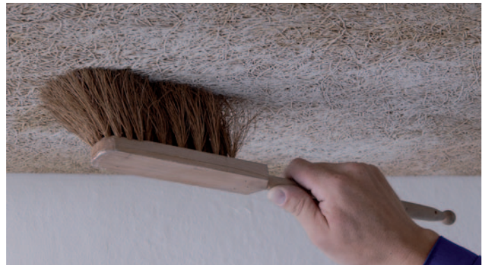
Brushing - Efflorescence, dust, etc. can be removed with a soft brush. Set loose fibres with a commercial grade acrylic primer.
