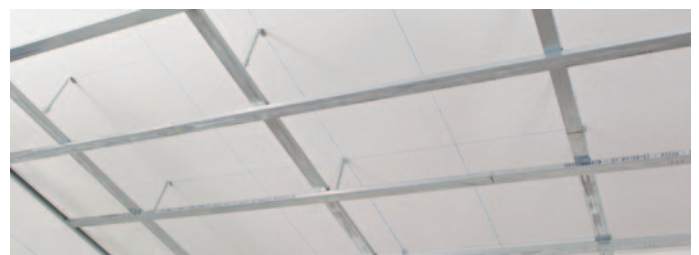
Finished ceiling grid.
