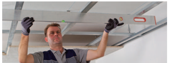
Aligning the Grid with a spirit level or laser level.
