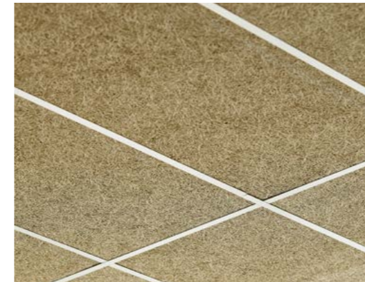
Lay In - Exposed Grid
