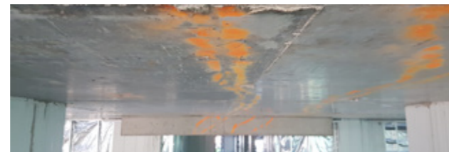
Formwork residue and concrete debris often present uneven fixing surfaces which are not made good prior to wall installation.
