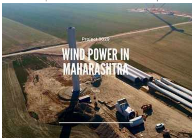
Project 3029: Wind Power in Maharashtra
