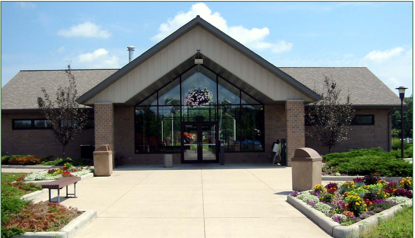
Photo Above: Juneau County Rest Area 10 Near Mauston.
