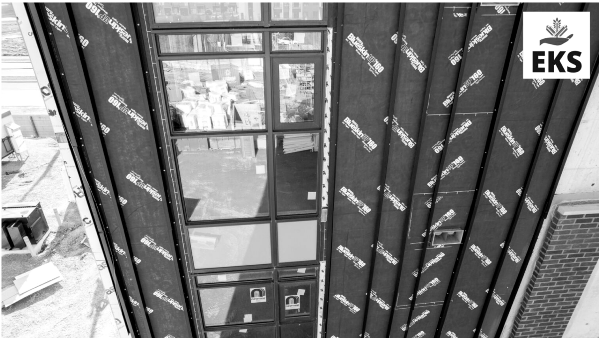
Figure 4 — Example vertical girt layout and glazing coordination.
