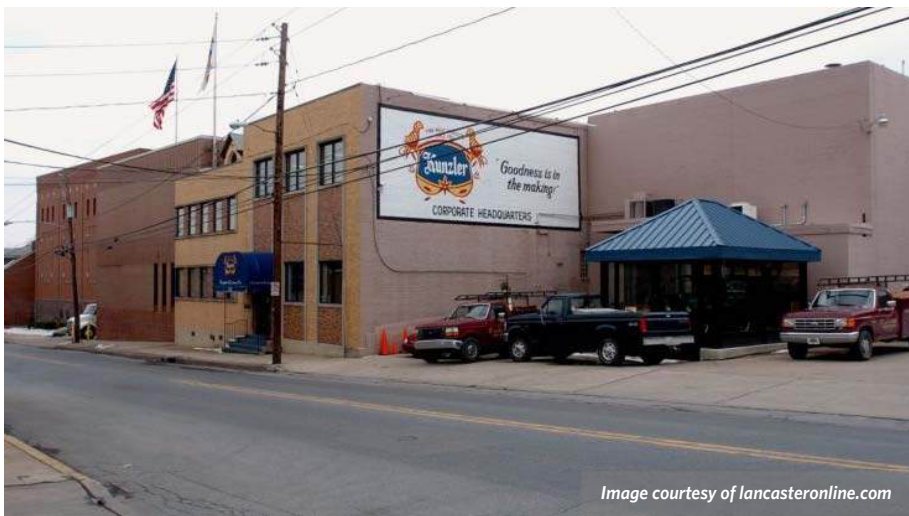
Figure 40: Kunzler and Company, located at 652 Manor Street.
