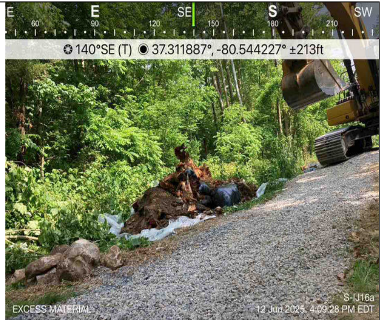
Photo Description: Stump and root system removed from bank.
