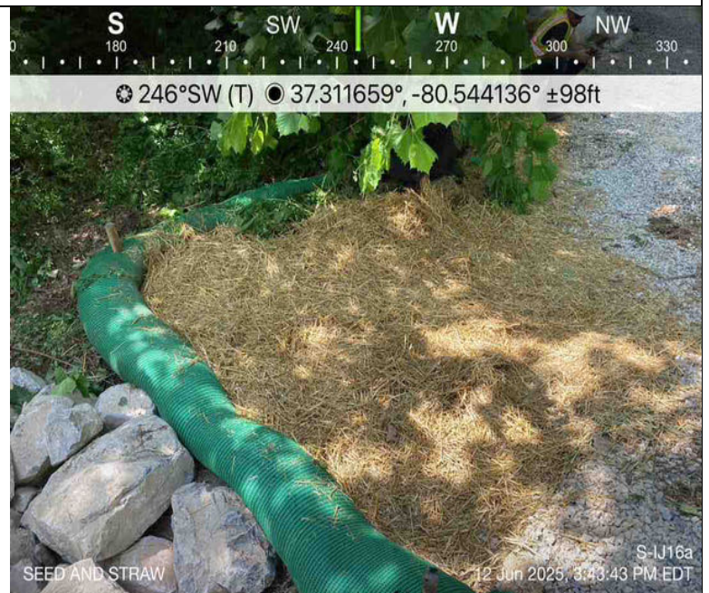
Photo Description: Stabilization applied to disturbed areas.
