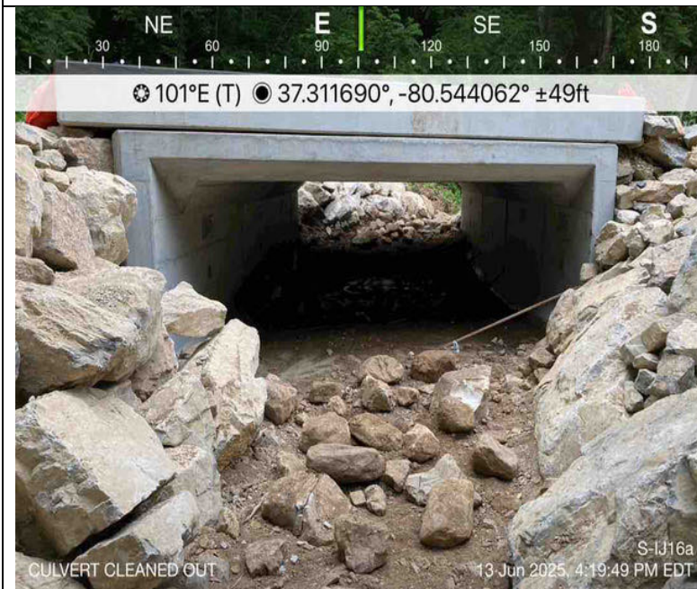
Photo Description: Culvert cleaned out of excess substrate.
