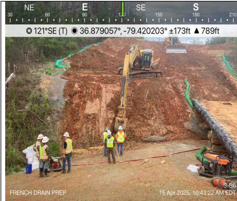
Photo Description: Laying back banks for French drain and rock armoring.
