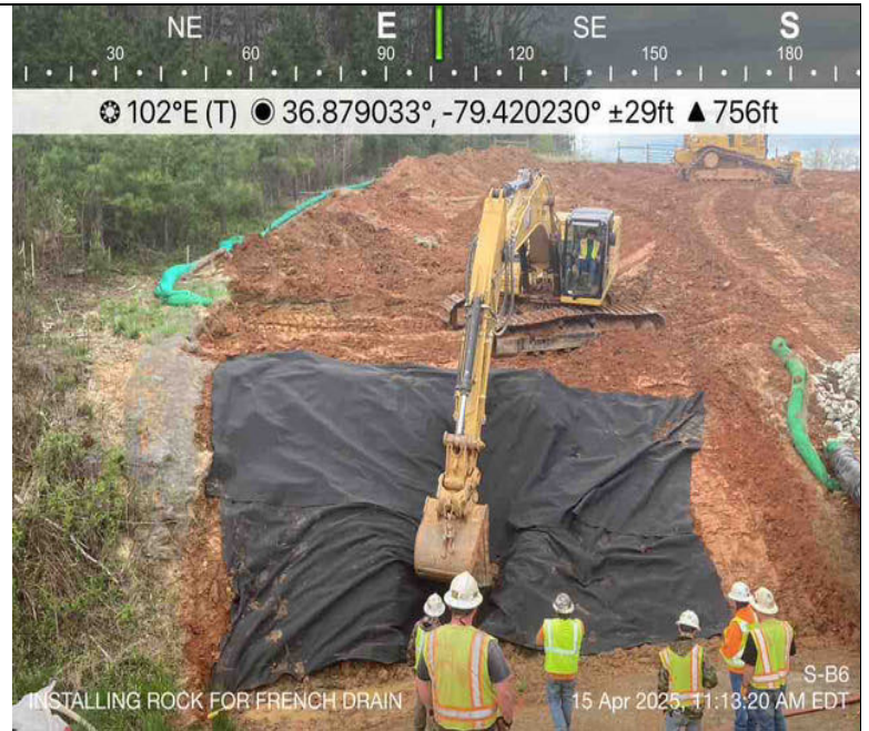
Photo Description: Installing geotech for French drain and rock armoring.
