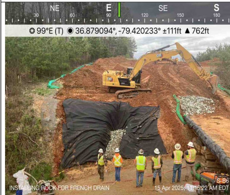
Photo Description: Rock installed for French drain.
