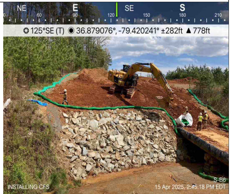
Photo Description: VDOT #2 installed over French drain for bank stabilization.
