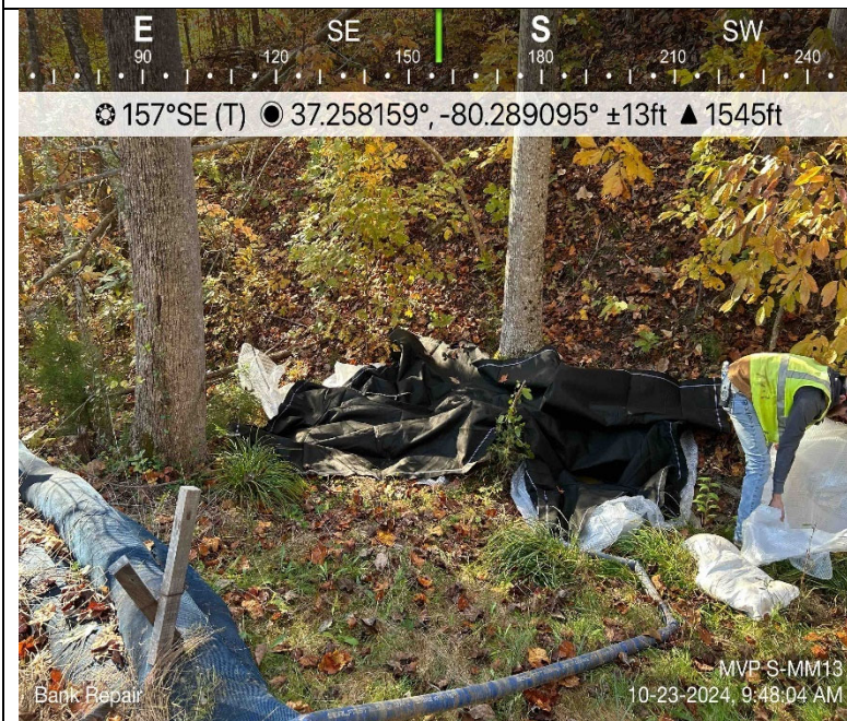
Photo Description: Downstream dam installed for bank repair.
