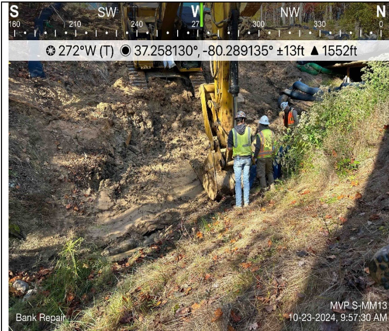
Photo Description: Bank repair underway within resource.
