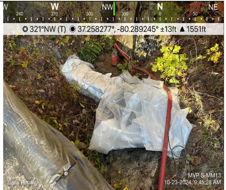
Photo Description: Upstream dam installed for bank repair
