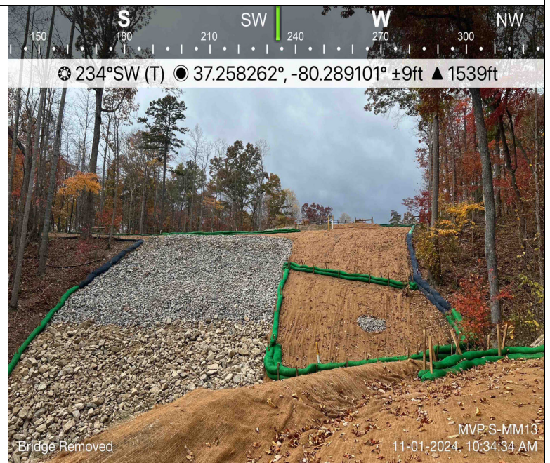
Photo Description: Overview of repaired slope.
