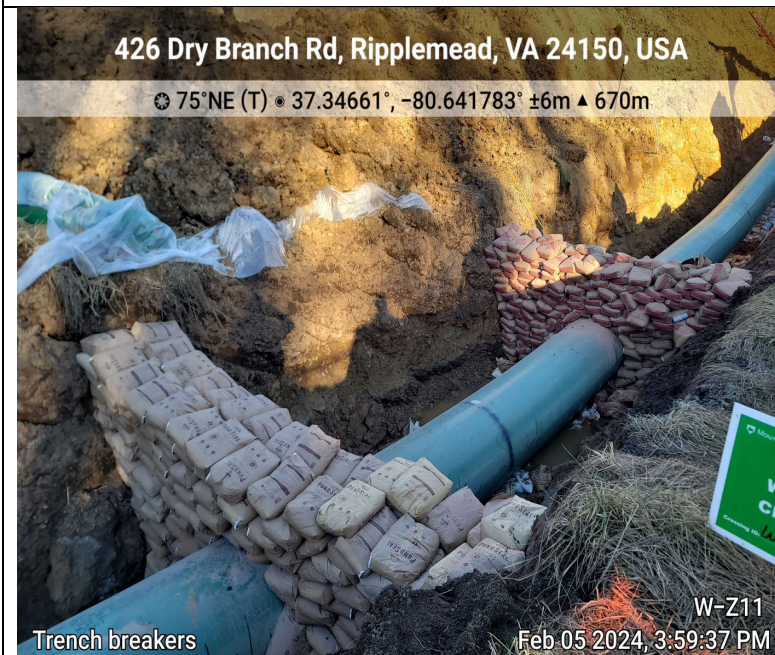
Photo Description: Trench breakers installed on both sides of resource.
