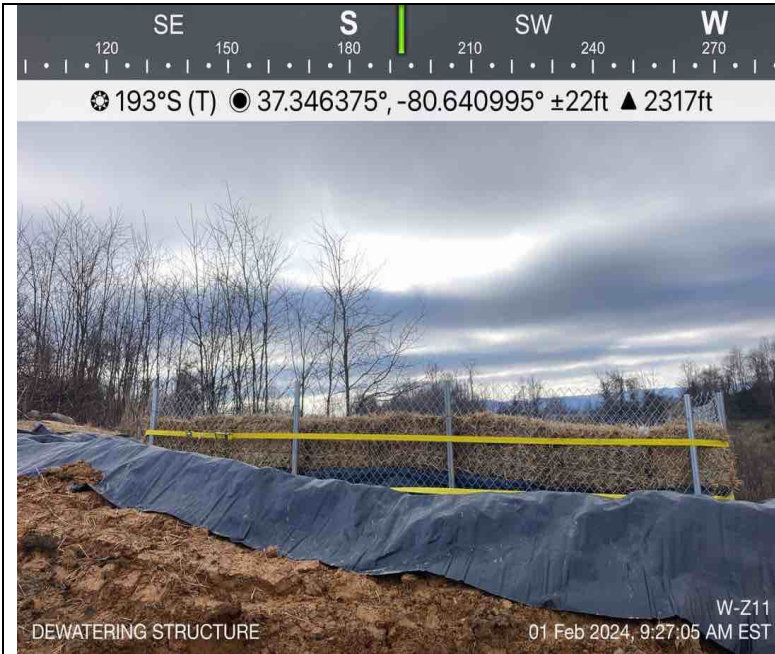
Photo Description: Dewatering structure installed for resource crossing.
