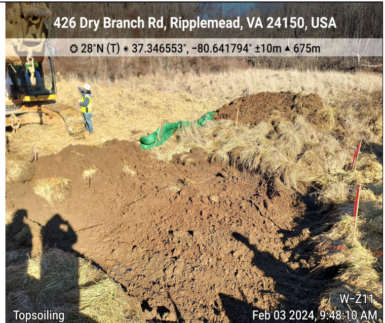
Photo Description: Topsoil removal and stockpiled separately from other soils.
