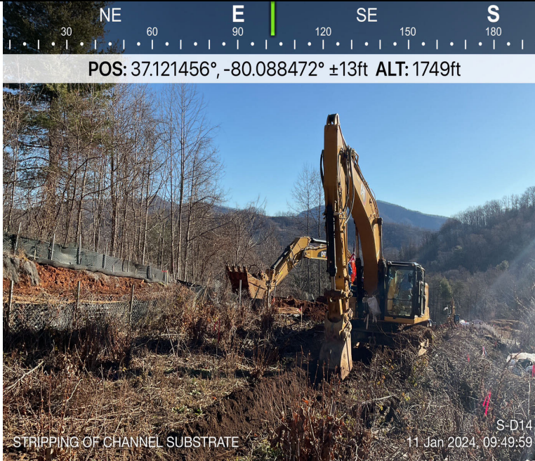
Photo Description: The channel substrate was stripped from the site.
