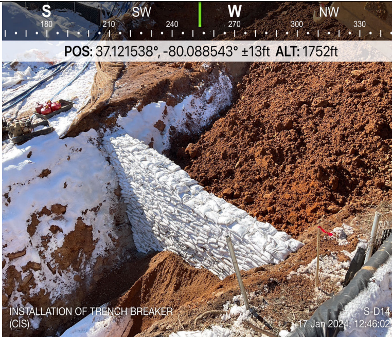
Photo Description: Installation of the impervious bentonite trench breaker (CIS).
