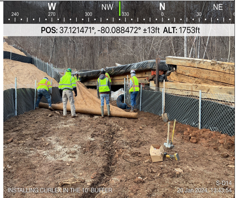
Photo Description: Curlex matting was installed within the 10-foot buffer zone.
