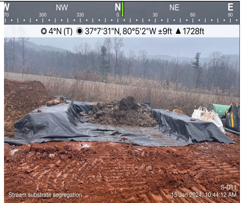
Photo Description: Stream substrate segregation in an upland area on timber mats and geotech. Substrate was stabilized with Kerlex.
