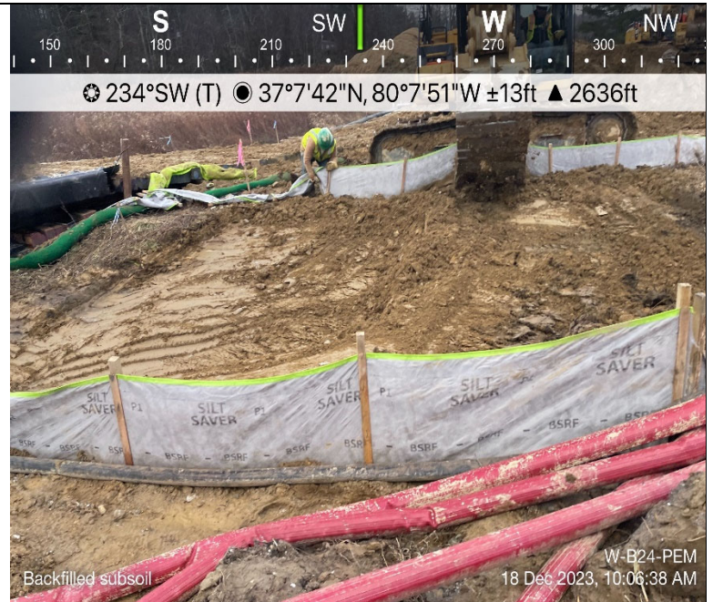
Photo Description: Subsoil backfill in wetland impact area.
