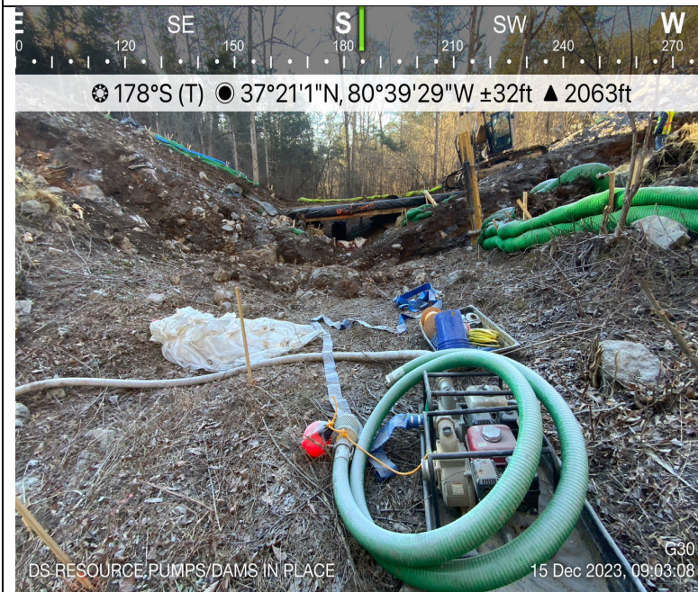
Photo Description: Dam and pumps in place.
