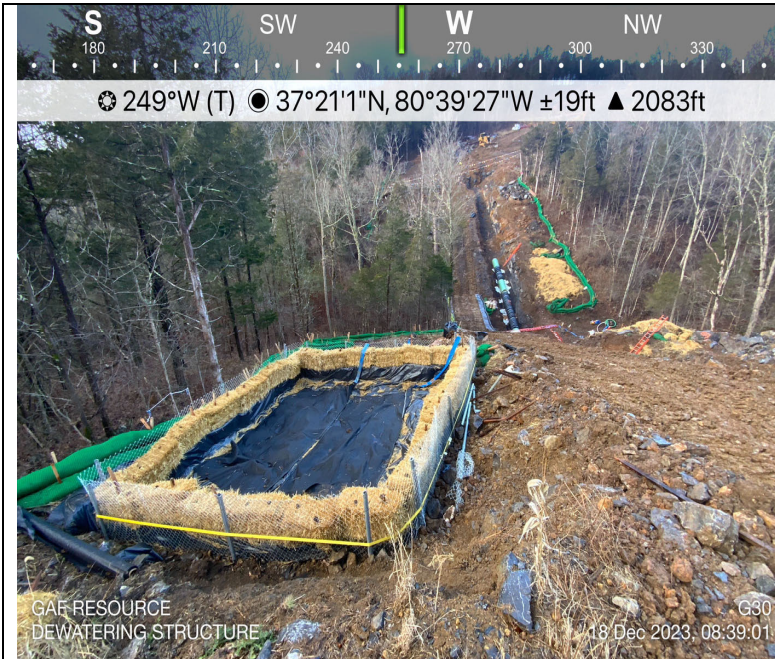
Photo Description: Dewatering structure located onsite.
