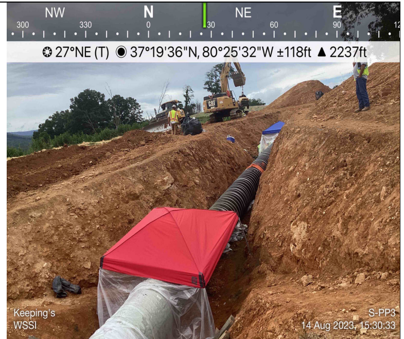
Photo Description: Keeping and coating at welds 2 and 3.
