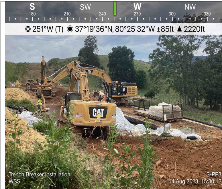
Photo Description: Trench breakers being installed.
