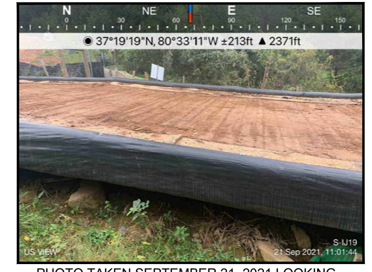
PHOTO TAKEN SEPTEMBER 21, 2021 LOOKING UPSTREAM FROM DOWNSTREAM IMPACT LIMITS
