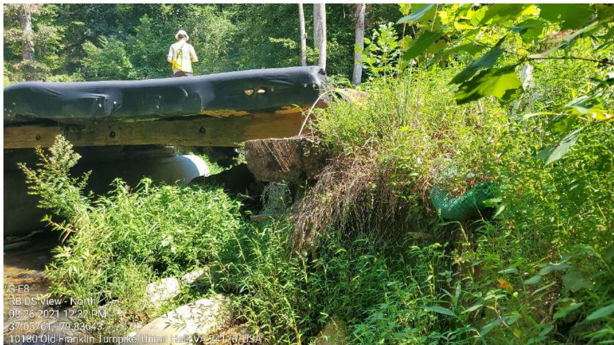
Photo Type: RB DS VIEW
