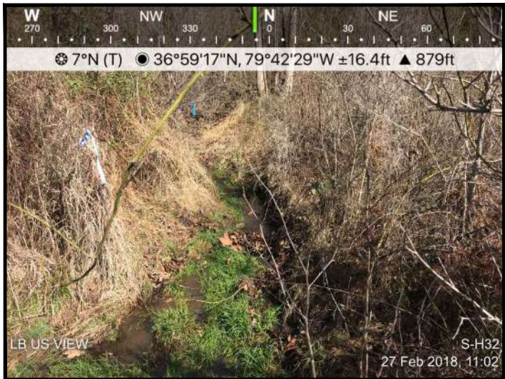
PHOTO TAKEN LOOKING UPSTREAM LEFT BANK ON 02/27/2018
